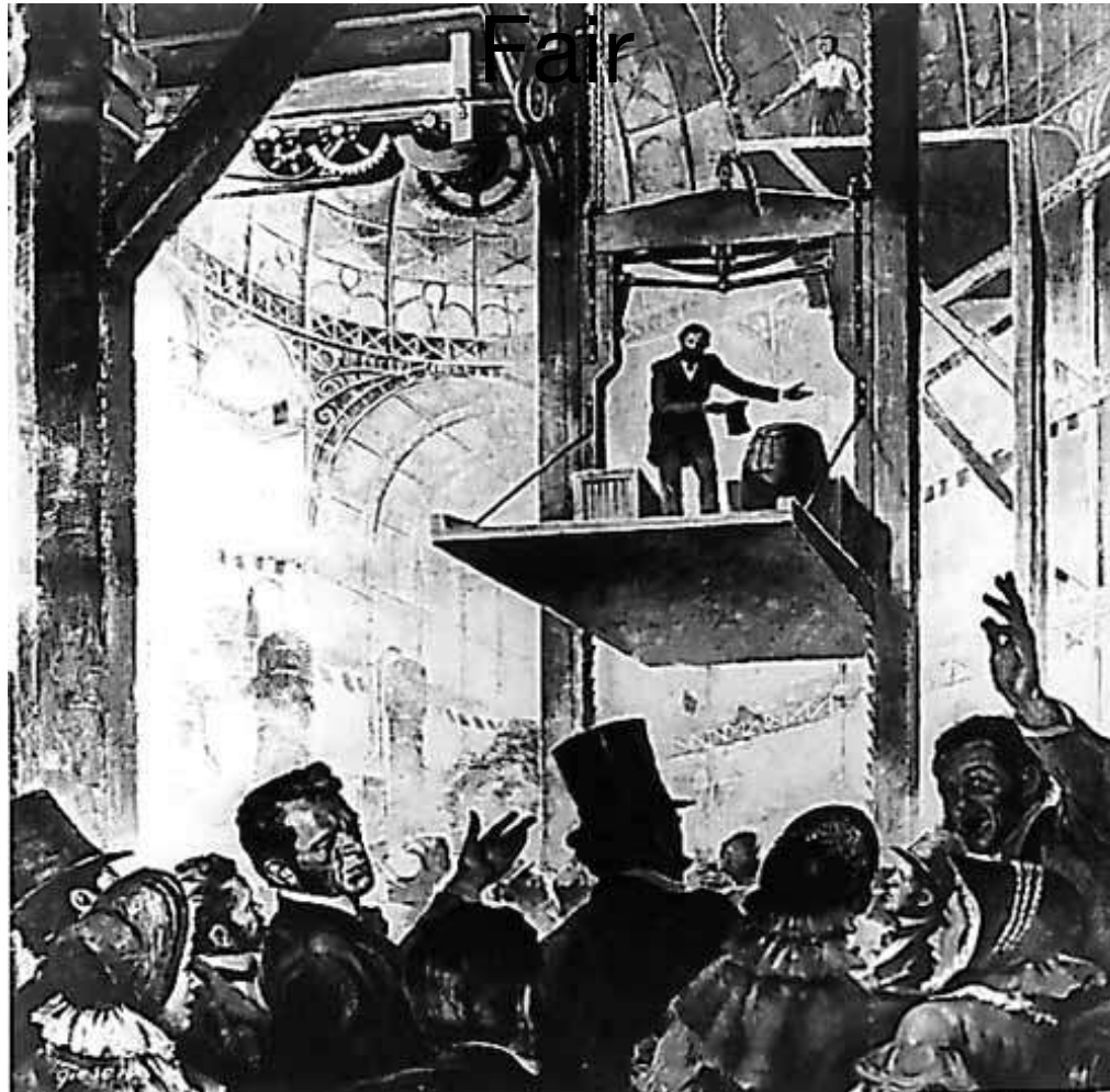
Otis stands on the elevator as the rope is cut.
